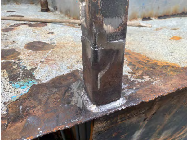
ITEM #12 Cropped Handrails Renewed
