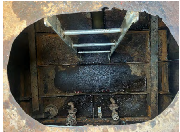
ITEM #10 Lazarette Sludge Cleaned
