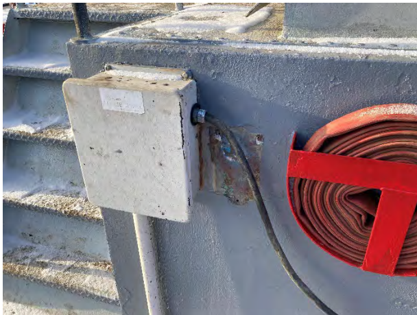
ITEM #19 Shore Power Cable Repaired
