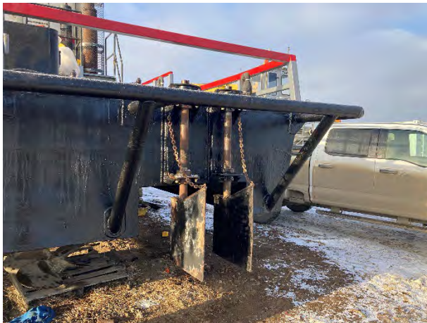
ITEM #35/36 Replaced Rudder Mounts and mounted Rudders
