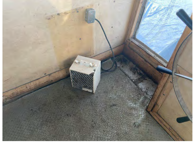
ITEM #39 Heater in Wheelhouse Replaced
