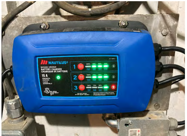
ITEM #31 House Battery Charger Replaced
