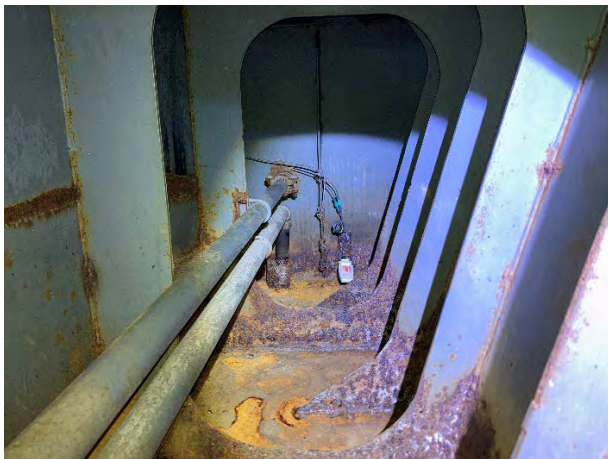
ITEM #9 Void space #3 Water and Sludge Cleaned
