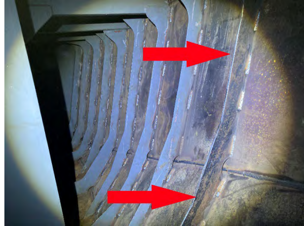
ITEM #4 Port Frame #20 Renewed
