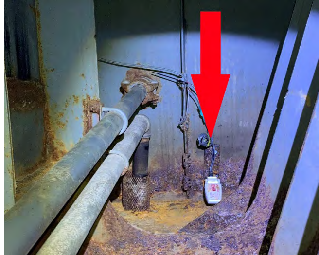
ITEM #6 Void Space #3 High water Sensor Secured
