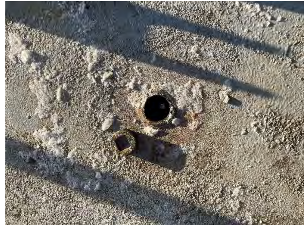
ITEM #16 Fuel Shut off Valves Made Functional
