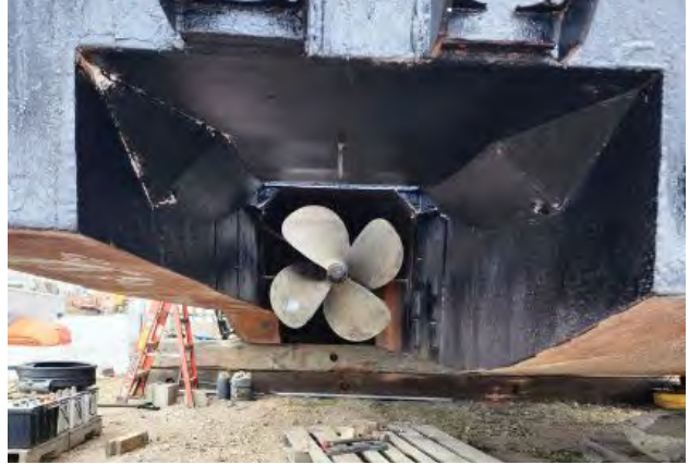
ITEM #32/33 Shafts and Props Installed Port
